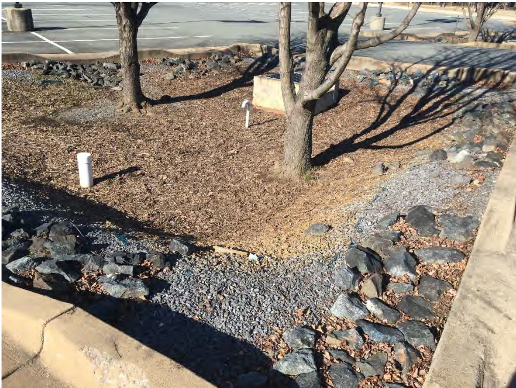
Overall, Facing North
