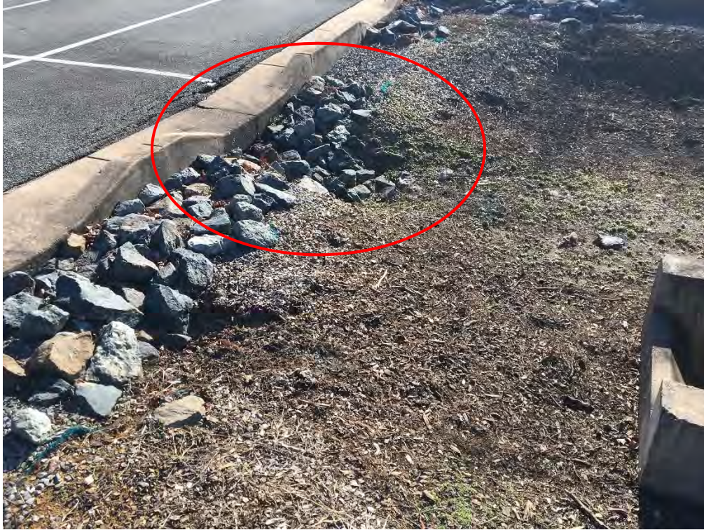
Erosion at inflow, water flows under curbing
