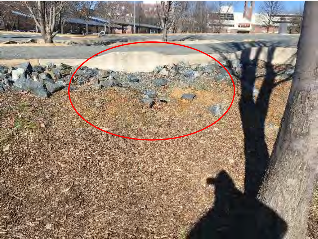
Erosion at Gravel Curtain - Facing North
