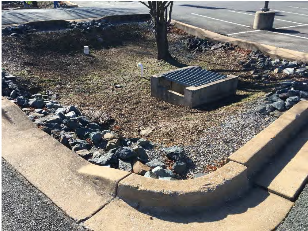
Overall, Overflow Device
